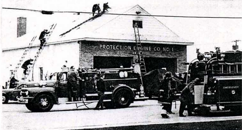
FIREHOUSE FIRE... Port's Volunteer Firemen responding to a general alarm on Tuesday, April 28th, at 6:34 a.m., for a fire at the Protection Engine Company No. 1 Annex on Channel Drive, may be seen above. Most of the damage occurred in the upstairs storage room where one of the 'racers' was completely gutted. (See front page photo also taken by Everitt J. Hehn)
