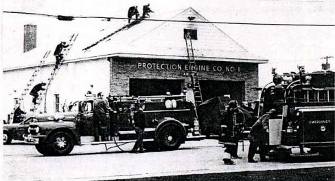
FIREHOUSE FIRE... Port's Volunteer Firemen responding to a general alarm on Tuesday, April 28th, at 6:34 a.m., for a fire at the Protection Engine Company No. 1 Annex on Channel Drive, may be seen above. Most of the damage occurred in the upstairs storage room where one of the 'racers' was completely gutted. (See front page photo also taken by Everitt J. Hehn)
